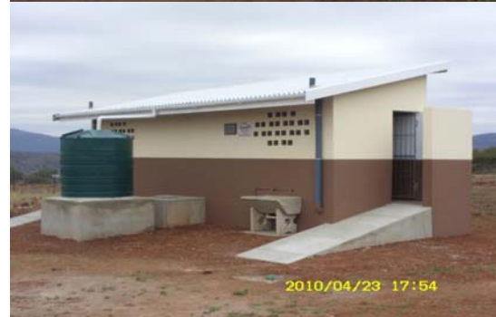
After building 3 classrooms , kitchen and an 8 cubicle toilet block at Ntabende Primary School.
